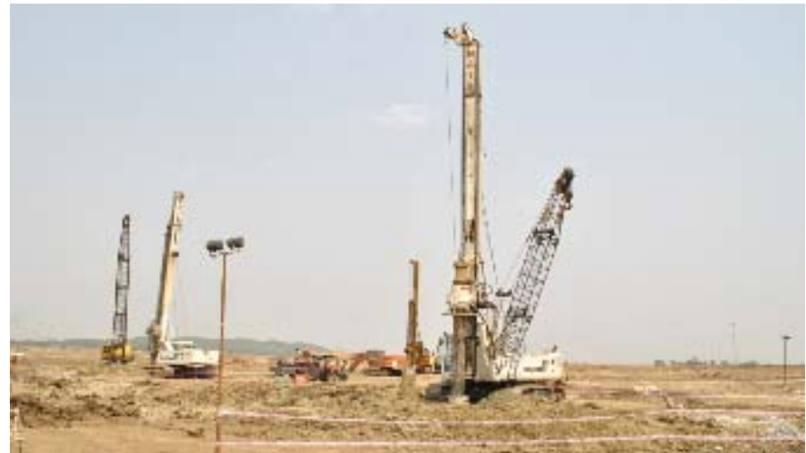
PILING WORK IN PROGRESS IN CONVERTER AREA
