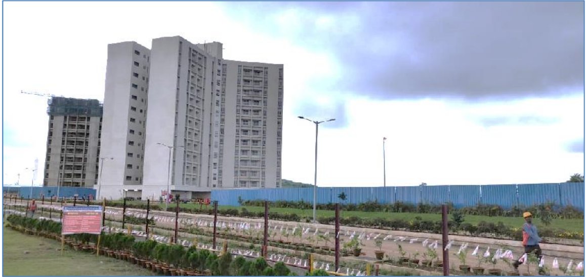
View of Township building
