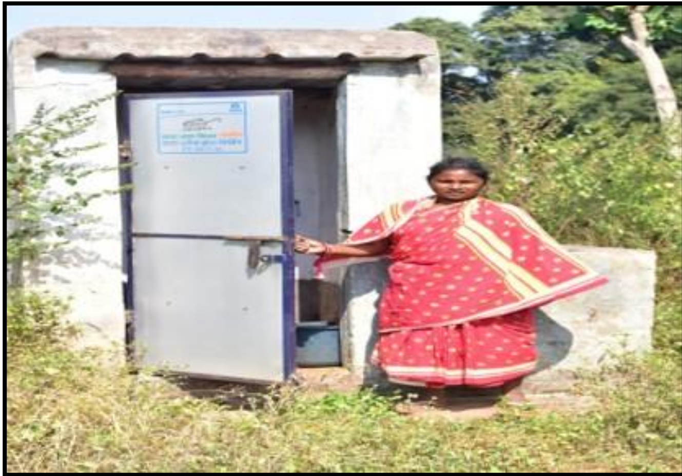
Photograph of toilet facility to individual household
