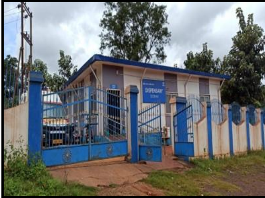
Photograph of dispensary at Deojhar GP
