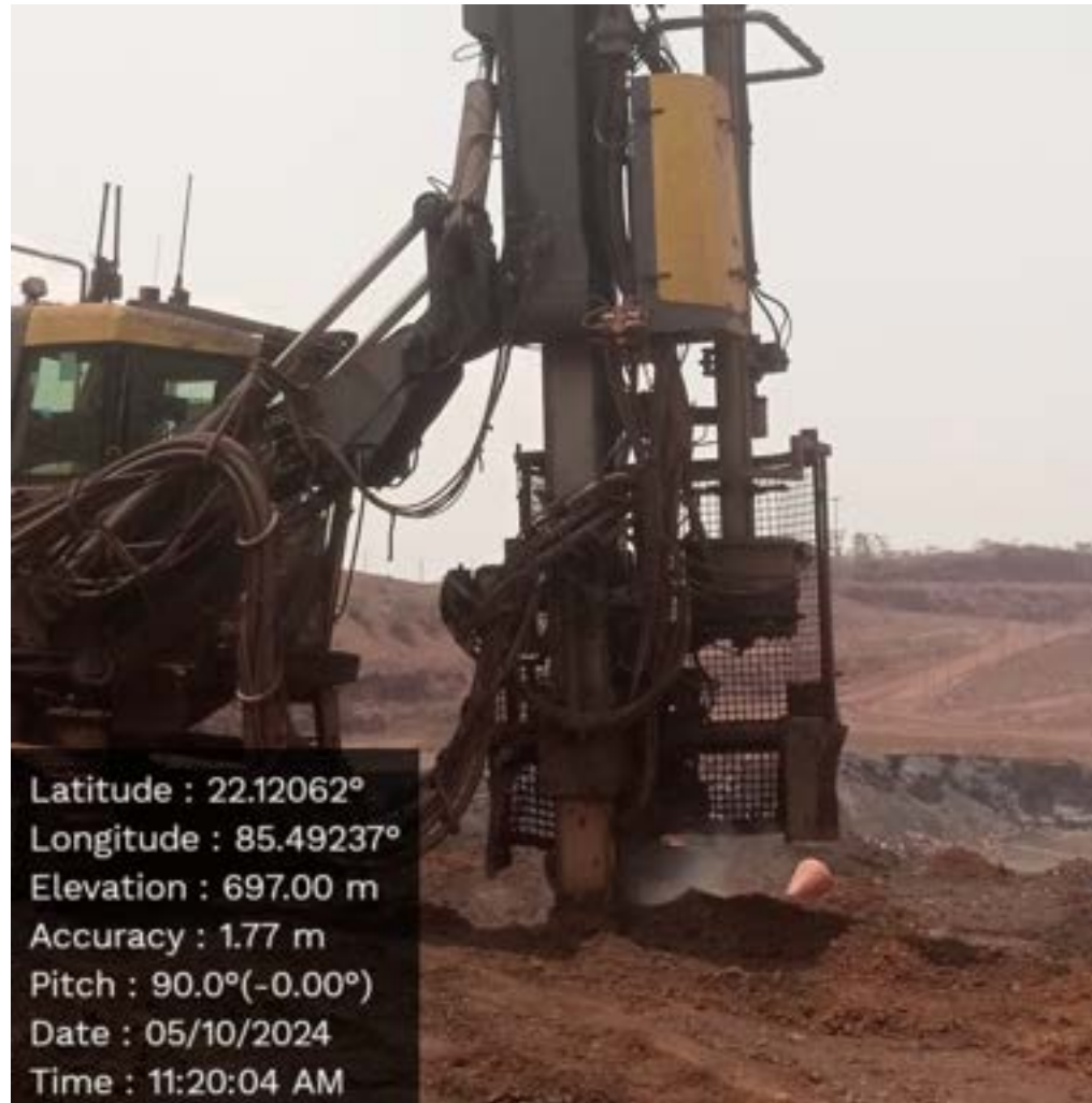
Drilling Machine Operation with water injection system
