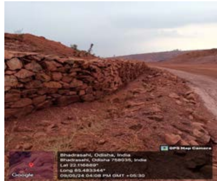
Garland Drain & retaining wall
