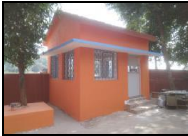
Photograph of Revamping of Murgamahadev Temple
