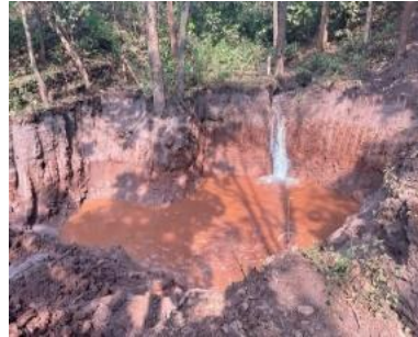
Fig 18: Garland Drains and Check Dams
