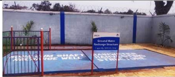
Fig 17: Rainwater Harvesting System at Khondbond Mine
