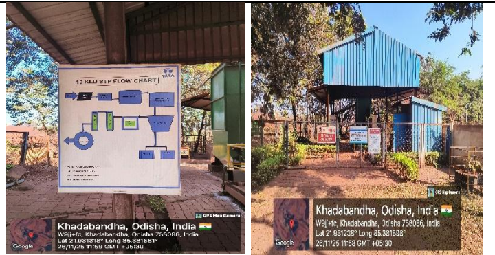
Fig 21: 10 KLD STP at Khondbond Iron and Manganese Mine
