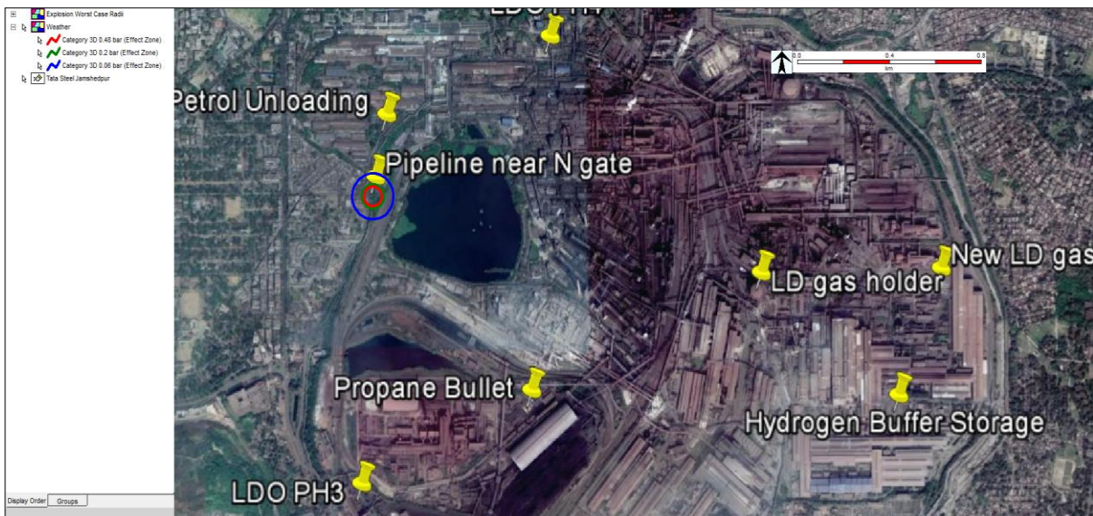
Figure 9.6: Explosion Overpressure for the release of H 2 from BF gas piping near N road gate
