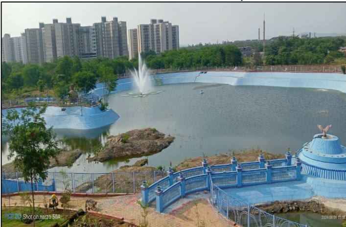
Rainwater Harvesting Pond
