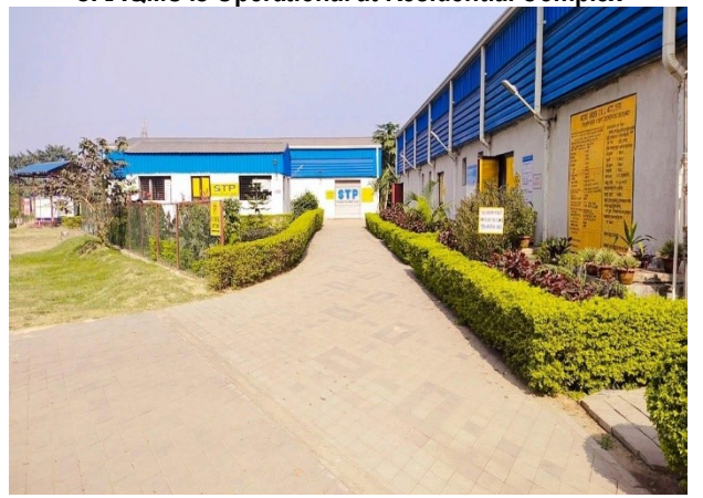
1000 KLD Sewage Treatment Plant in operation
