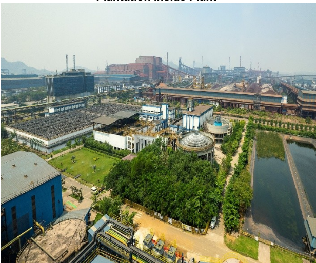
Roof Top Solar panel and Miyawaki Plantation at TWTP
