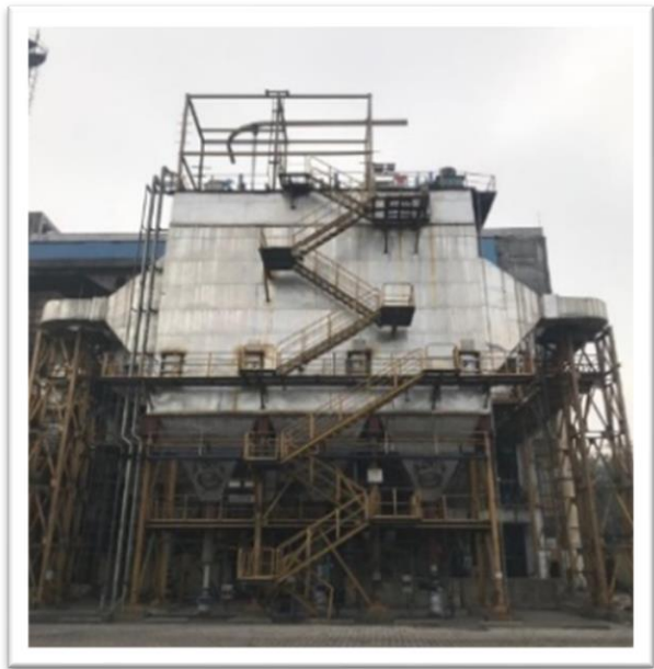
Electrostatic Precipitator (ESPs) at Boiler Stack
