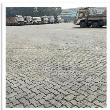
Paver Blocks on loose soil
