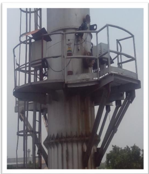
Continuous Emission Monitoring System at Boiler Stack (CEMS)
