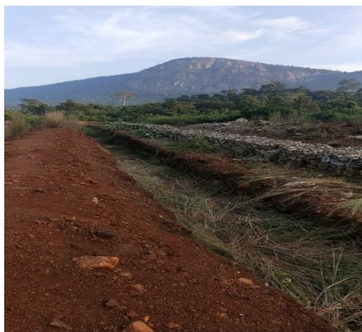
Garland drain with retaining wall cleaned
