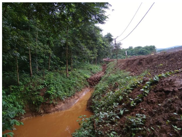
Garland drain with settling pin & Check dam
