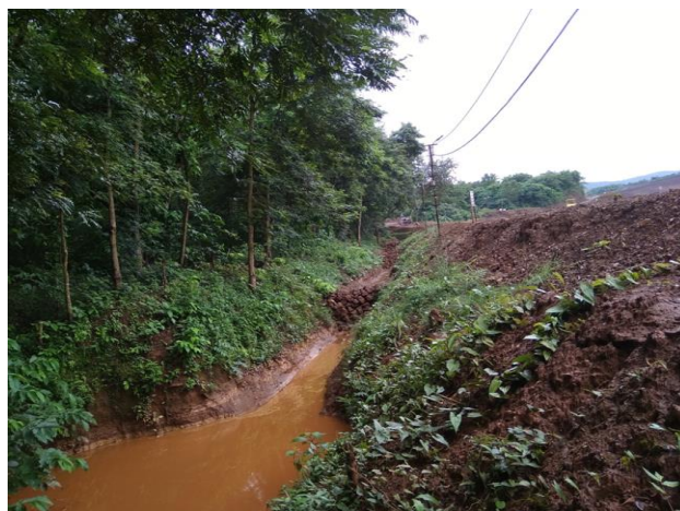
Garland drain with settling pin & Check dam
