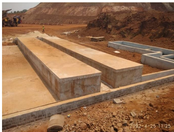
Vehicle washing with Oil & Grease separation pit
