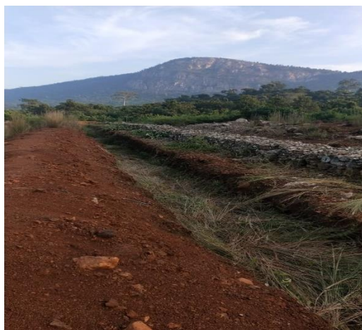
Garland drain with retaining wall cleaned
