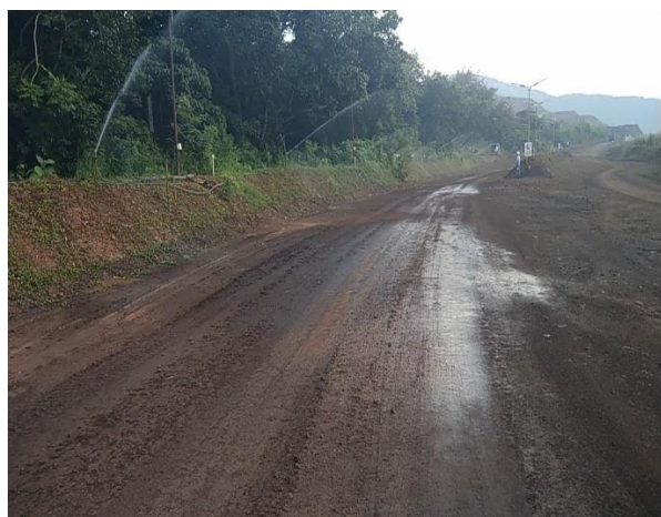
Mines haul road water sprinkling
