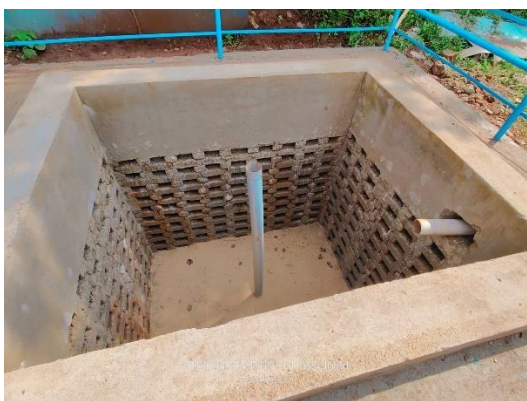
Roof top Rainwater Harvesting Structures constructed for Ground Water Recharge
