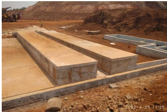
Vehicle washing with Oil & Grease separation pit
