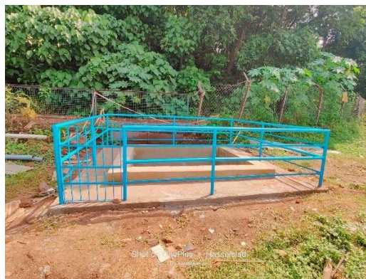
Roof top Rainwater Harvesting Structures constructed for Ground Water Recharge
