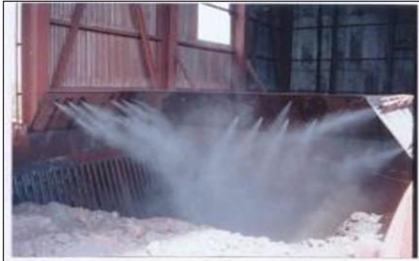
Dry fog systems at dump hoppers
