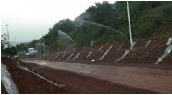
Use of fixed water sprinklers at haul roads for dust suppression
