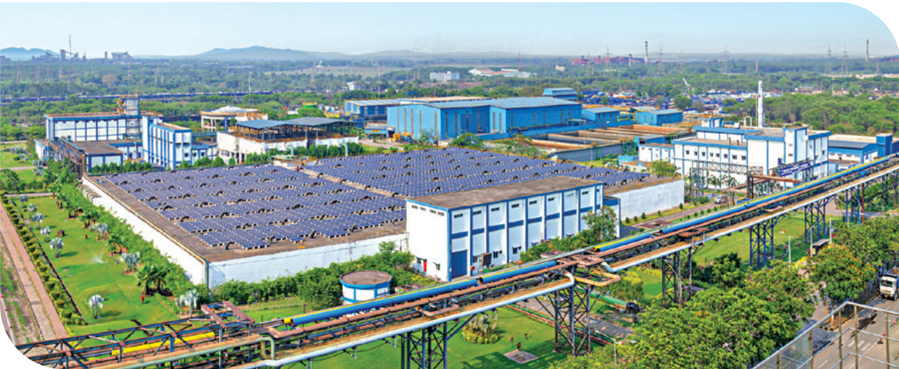
Solar Panels, WTP Building, Kalinganagar
