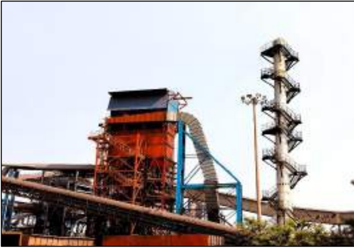
Installation of New Bag Filter at MBF-2 RMHs
