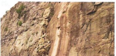
Fig.2: Plane failure
