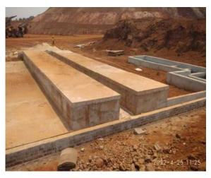
Vehicle washing with Oil & Grease separation pit
