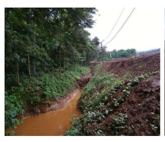
Garland drain with settling pin & Check dam
