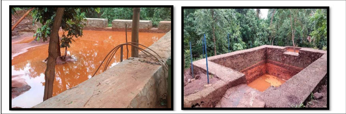
Settling Pond and settling cum percolation pond developed
