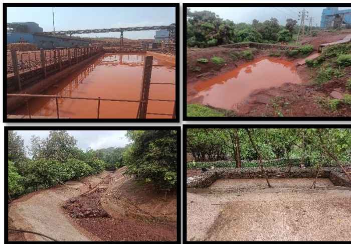
Siltation pond and catch drains in iron mines area
