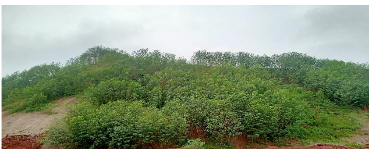
Coir Matt at Sub Grade dumps
