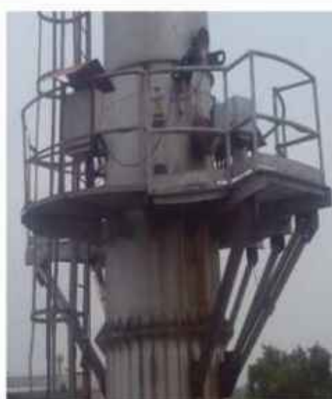
Continuous Emission Monitoring System at Boiler Stack (CEMS)
