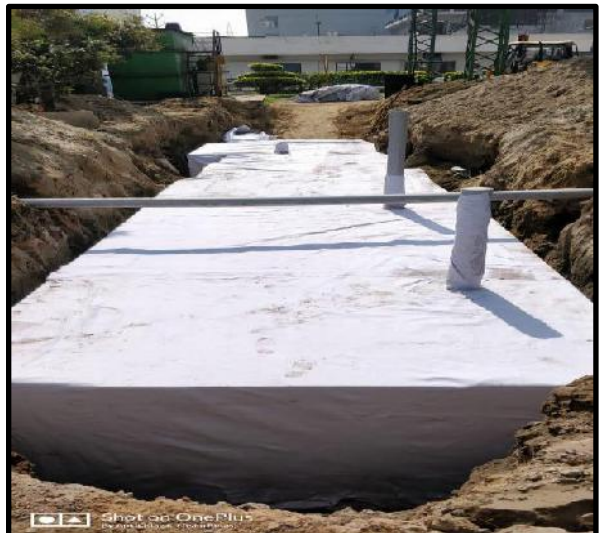
GEOTEXTILE COVERING
