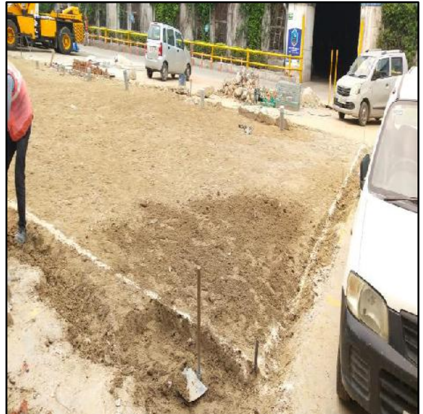
BACK FILLED AFTER INSTALLATION
