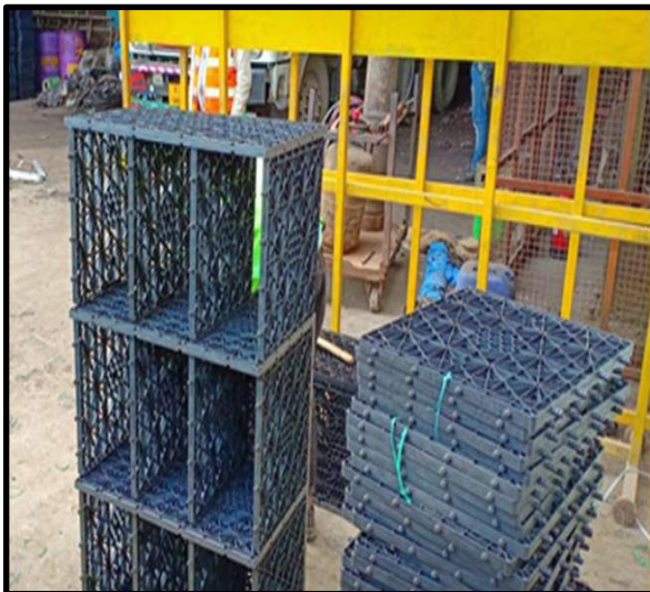
RAINMAXX MODULE ASSEMBLY
