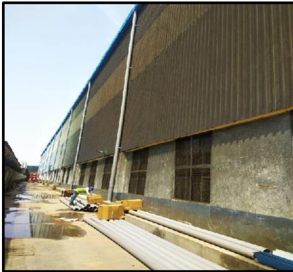
DOWNTAKE PIPES CONNECTION
