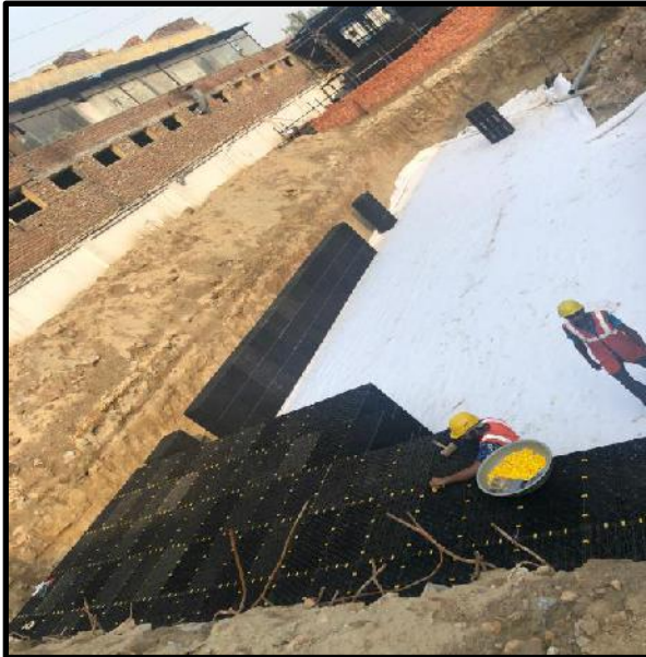
RAINMAXX MODULE ASSEMBLY
