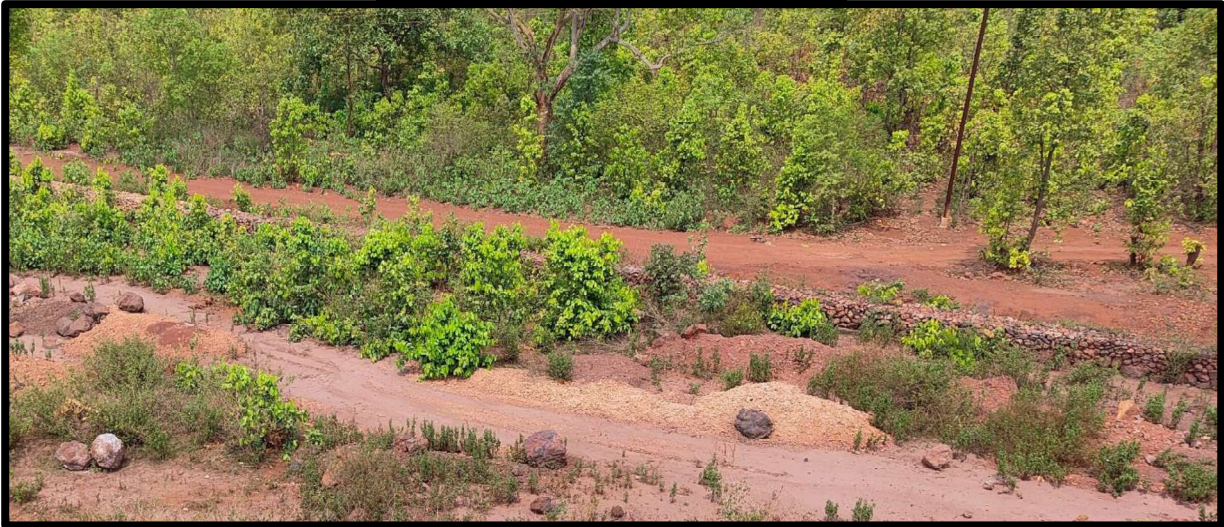
Garland Drains, & Retaining walls
