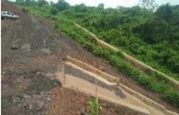
Fig.3 & 4 Rain Passes for slope protection
