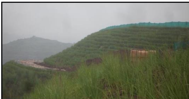
Fig.5 Coir Matting of Dump Slopes for stabilization
