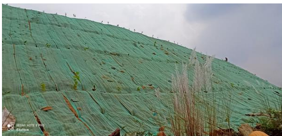
Fig.5 Coir Matting of Dump Slopes for stabilization
