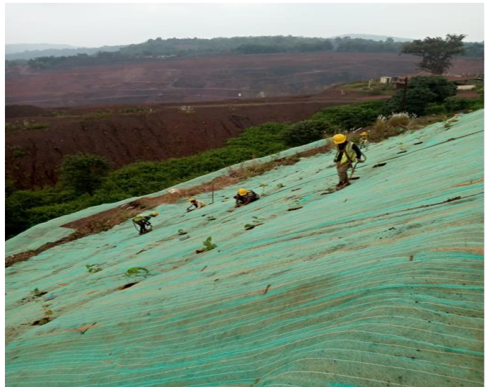
Fig.5 Coir Matting of Dump Slopes for stabilization
