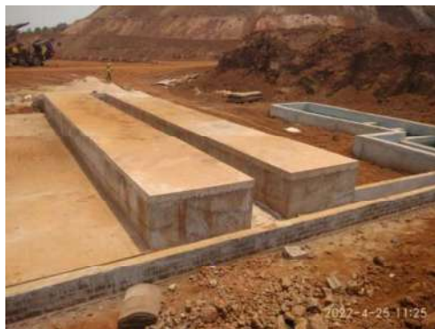
Vehicle washing with Oil & Grease separation pit
