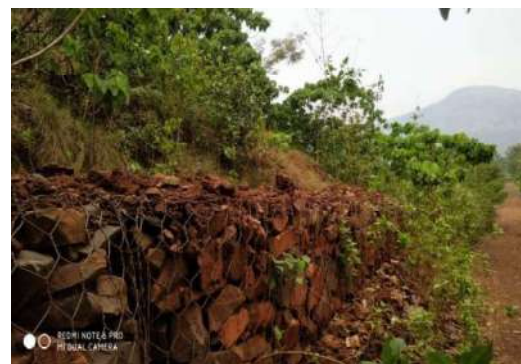
Waste dump management with Retaining wall and Garland drain construction
