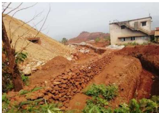
Waste dump management with Retaining wall and Garland drain construction
