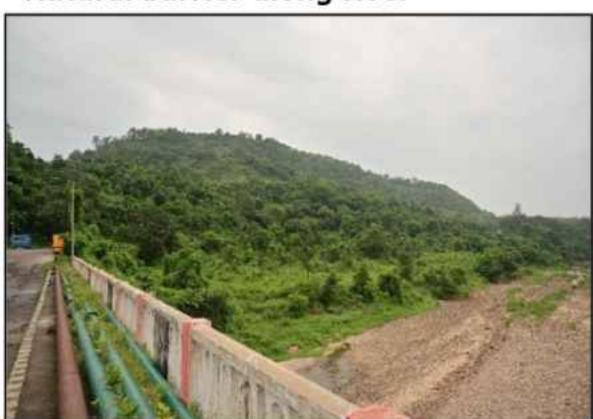
Embankment constructed by using OB which is stabilized and covered with greenery
