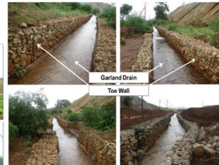
Garland Drains & Toe Walls
