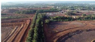
Back filling of mined out ore body II. It is planned to accumulate ~ 300 lakh cum of overburden which will save 60 Ha of land from degradation
