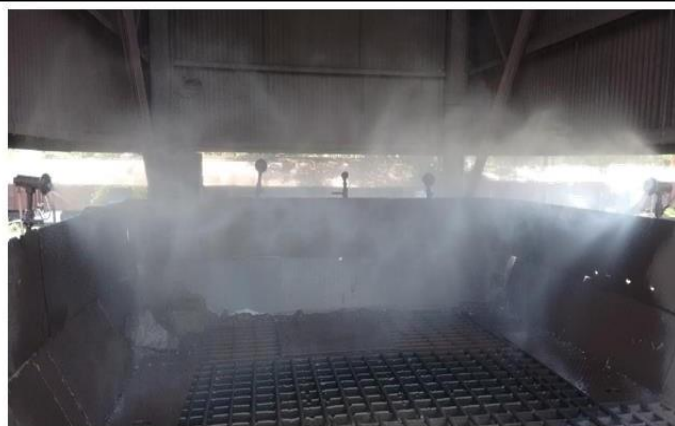
Dry Fogging System for Fugitive dust suppression
