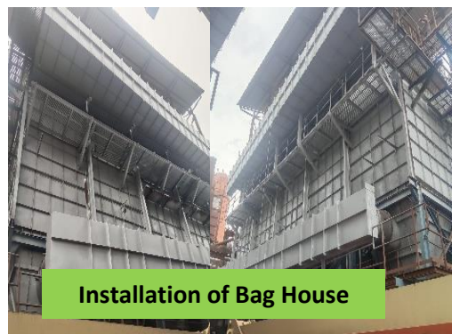
DHS connected to separate bag filter.
