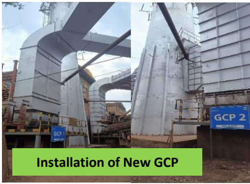
DHS connected to separate bag filter.
