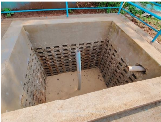
Roof top Rainwater Harvesting Structures constructed for Ground Water Recharge
