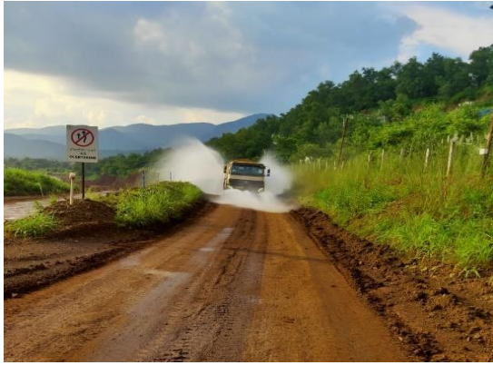
Water sprinkling through movable water tanker & Fixed Sprinkler
