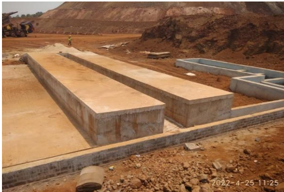
Vehicle washing with Oil & Grease separation pit
