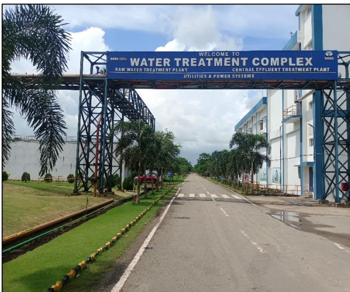
Water Treatment Complex at TSK
