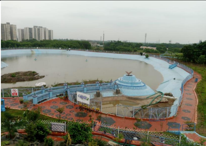
Rainwater Harvesting Structure
