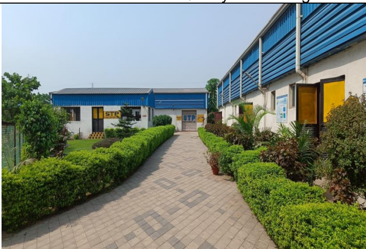
(1000 KLD) STP is in Operation
