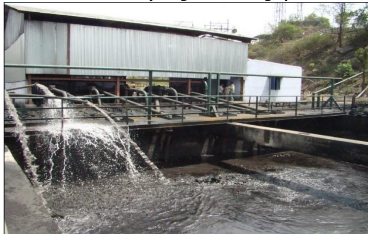
Water Recycling from tailings ponds
