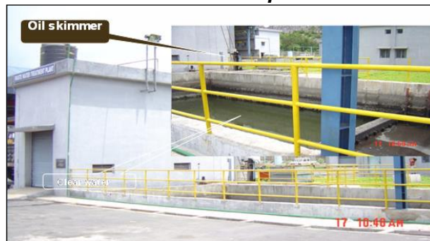
Oil & Grease trap at mines
