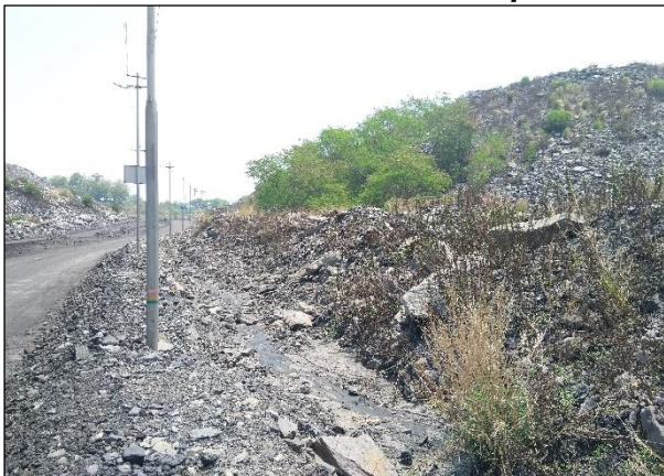
Catch Drains at the toe of dumps
