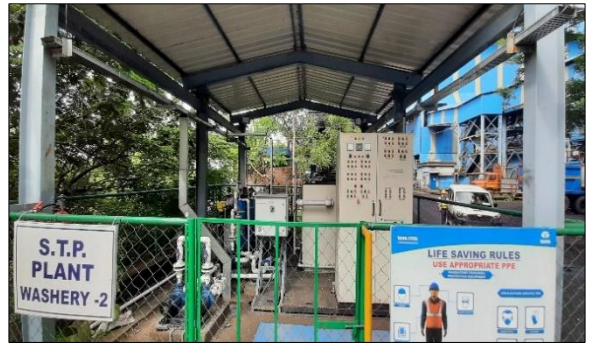
100 KLD STP at Chainpur
