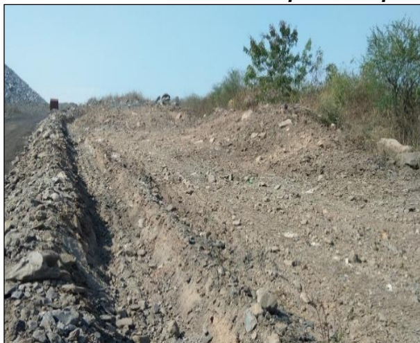
Maintained catch drain of Topsoil Dump
