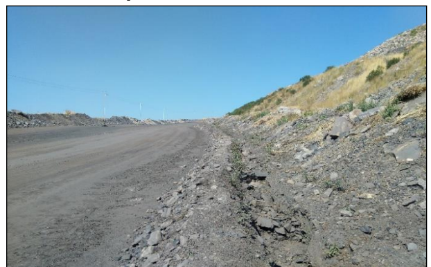
Catch Drains at the toe of dumps
