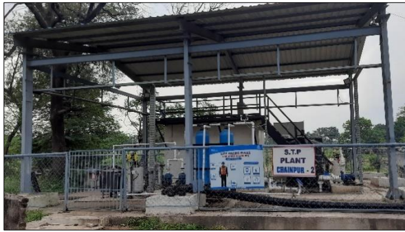
5 KLD STP at Washery-3 Canteen
