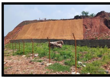
Back filling of quarry by Over Burden
