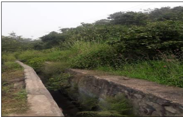
Catch Drains at the toe of dumps
