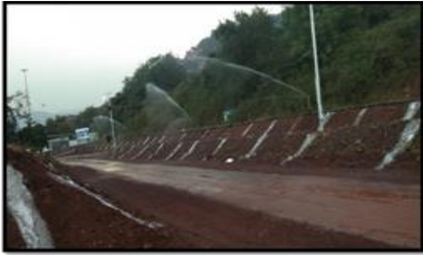
FIXED WATER SPRINKLER
