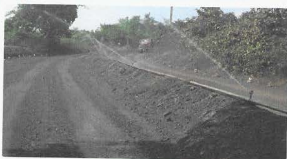
Fixed Sprinkling System
