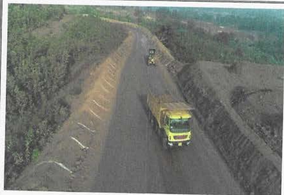
Haul Road with Safety Berms
