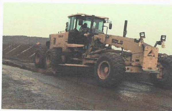
Grader for Haul Road
