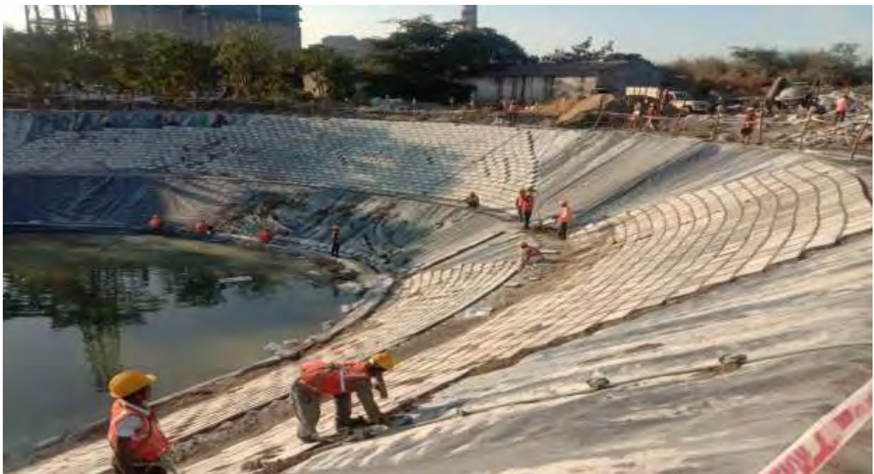
Photo – 3: Photo Showing the Pitching of Sidewalls of the Pond
