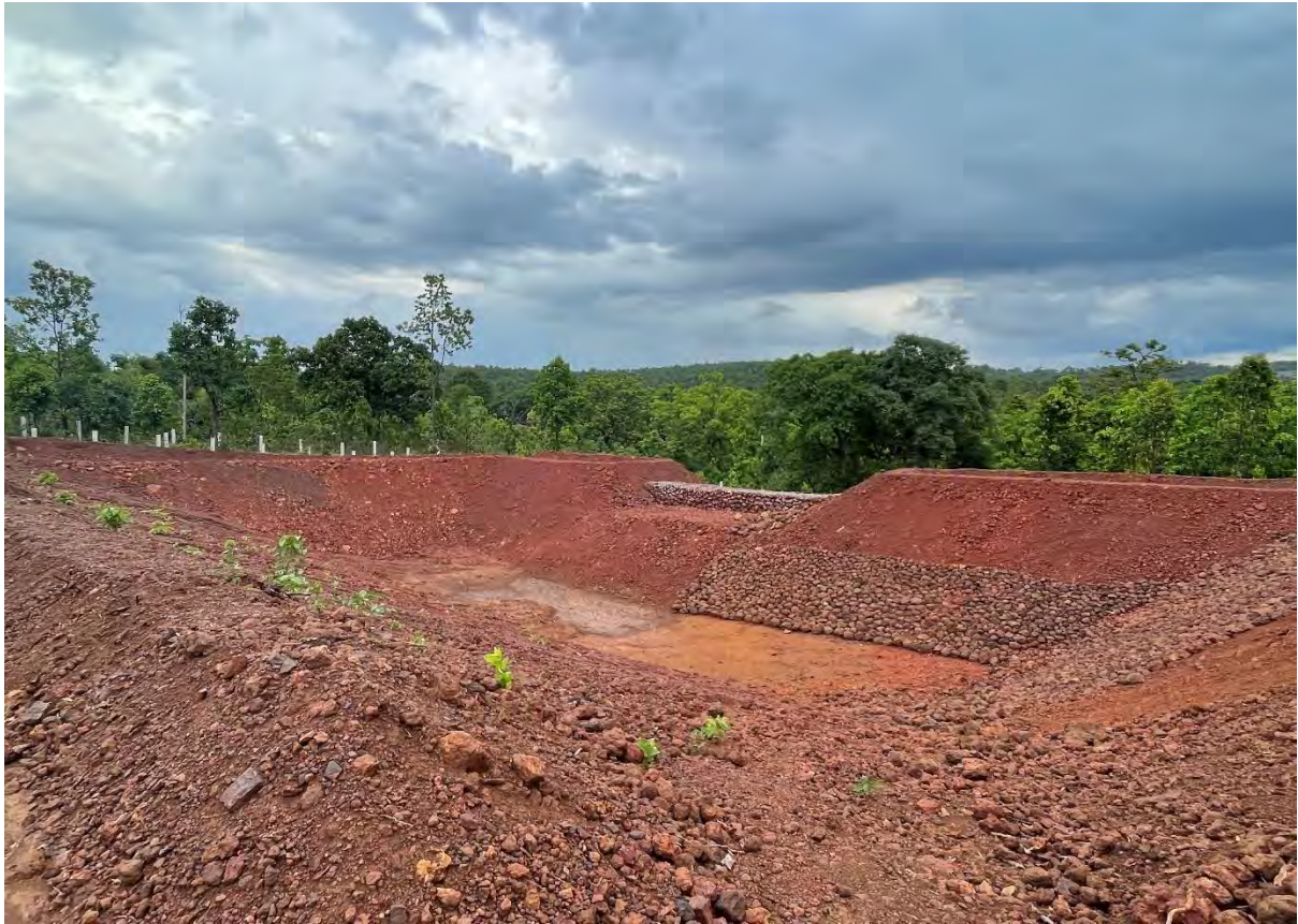
Photo 2- Retaining wall & garland drain near Mineral Stackyard
