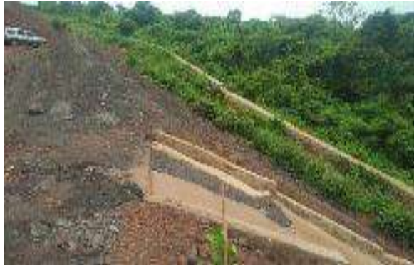
Fig.3 & 4 Rain Passes for slope protection
