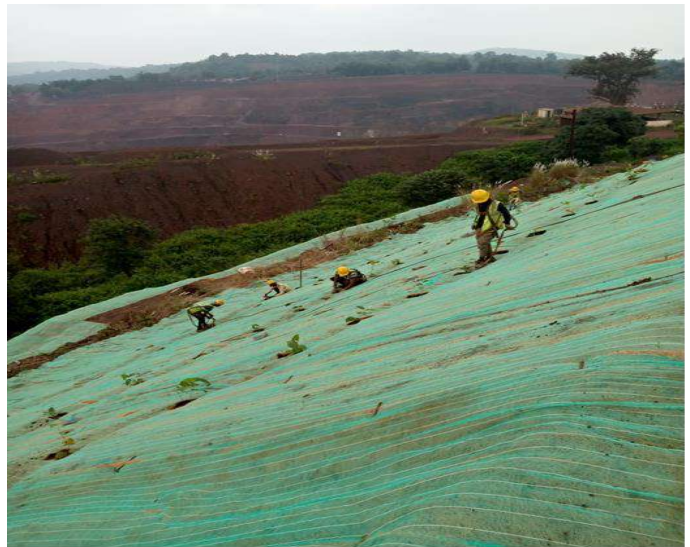
Fig.5 Coir Matting of Dump Slopes for stabilization
