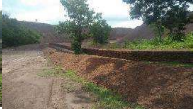
Fig.2 Garland Drain with Toe Wall
