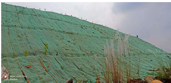
Fig.5 Coir Matting of Dump Slopes for stabilization
