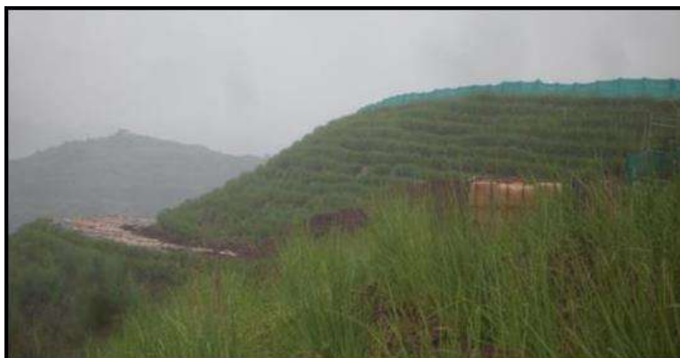
Fig.5 Coir Matting of Dump Slopes for stabilization
