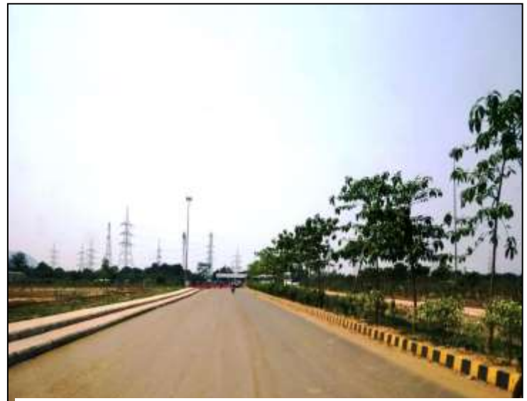
Metaled roads inside plant premises with separate path for bi-cycle
