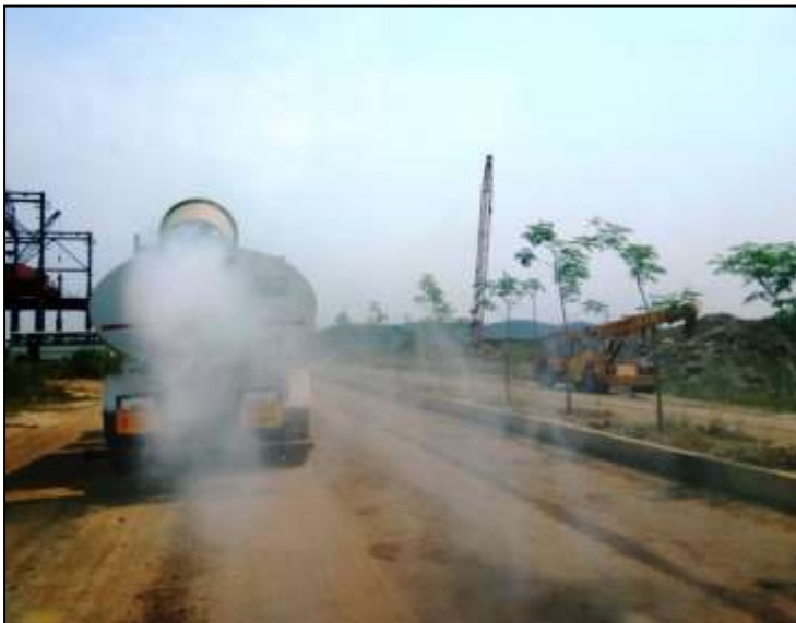
Water sprinkling on internal roads through mist type sprinkler
