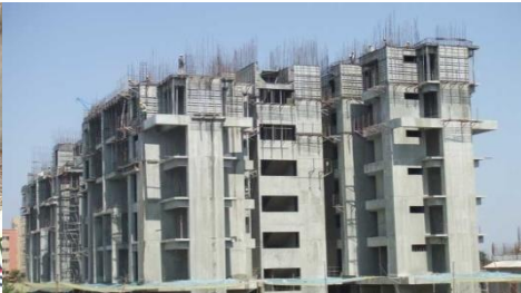
With modern formwork –Walls
