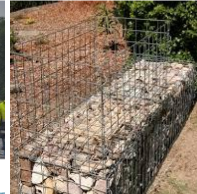
Gabions – Stone walls
