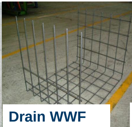
Open loop Stirrup Cage for Beam
