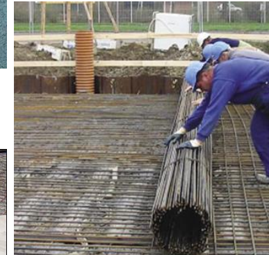
Metros – Higher dia F- WWF or Carpet reinforcement
