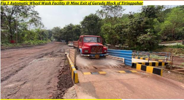
Fig.2 Automatic Wheel Wash Facility @ Guruda Block of Tiringpahar
