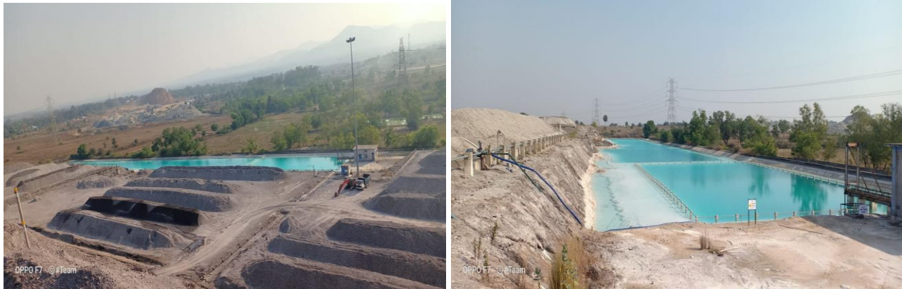
Rain Water Harvesting Pond
