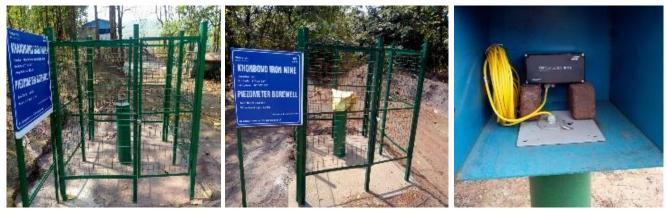
Piezometer (STP and Manganese) with digital recorder
