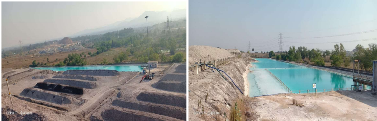
Rain Water Harvesting Pond
