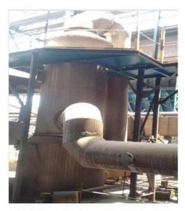
Fume Extraction System For existing Plant
