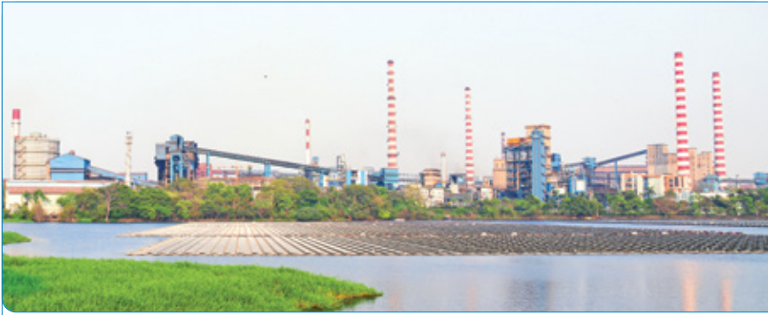
Solar panels installed at the cooling pond, Tata Steel Jamshedpur
