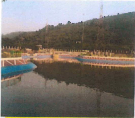
New Rain water Harvesting structure
