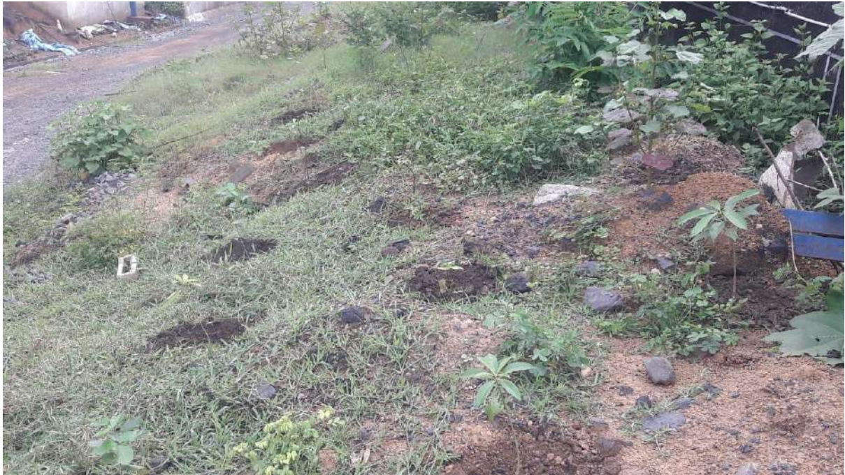
Picture: Plantation around some patches of the boundary wall of washery (JCPP) during this monsoon season.
