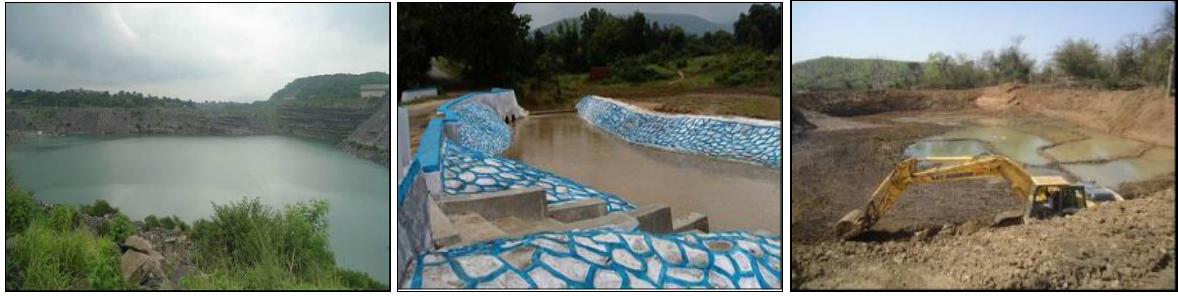
Rainwater harvesting structures
