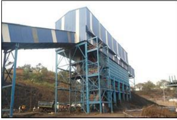
Coal transport by conveyor belt
