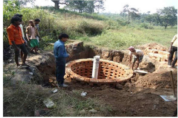
Artificial ground water recharge pit (Bore well) in Birlor village
