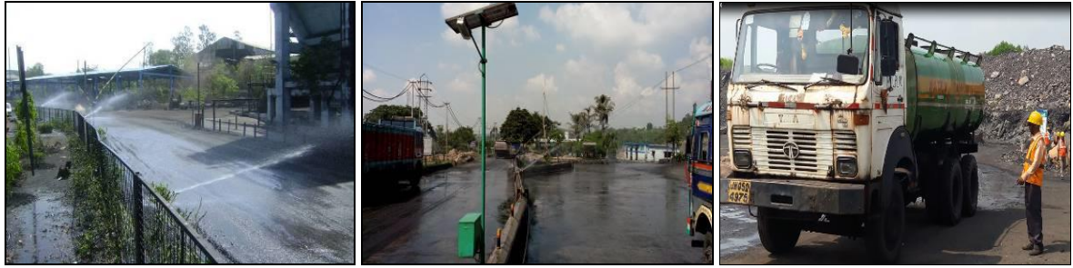
Use of Fixed & mobile water sprinklers in area
