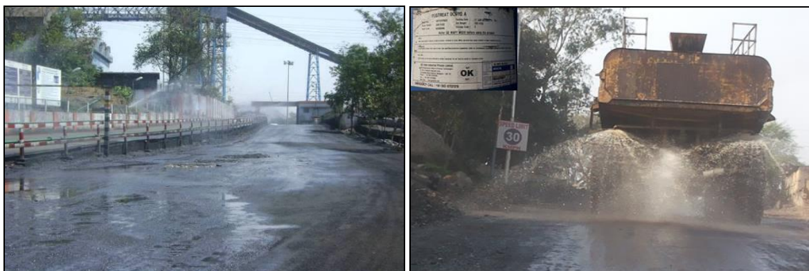
Fixed and mobile water suppression system
