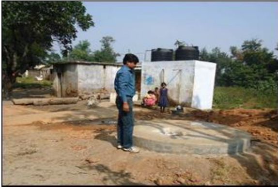
Artificial ground water recharge pit (Bore well) in Birlor village
