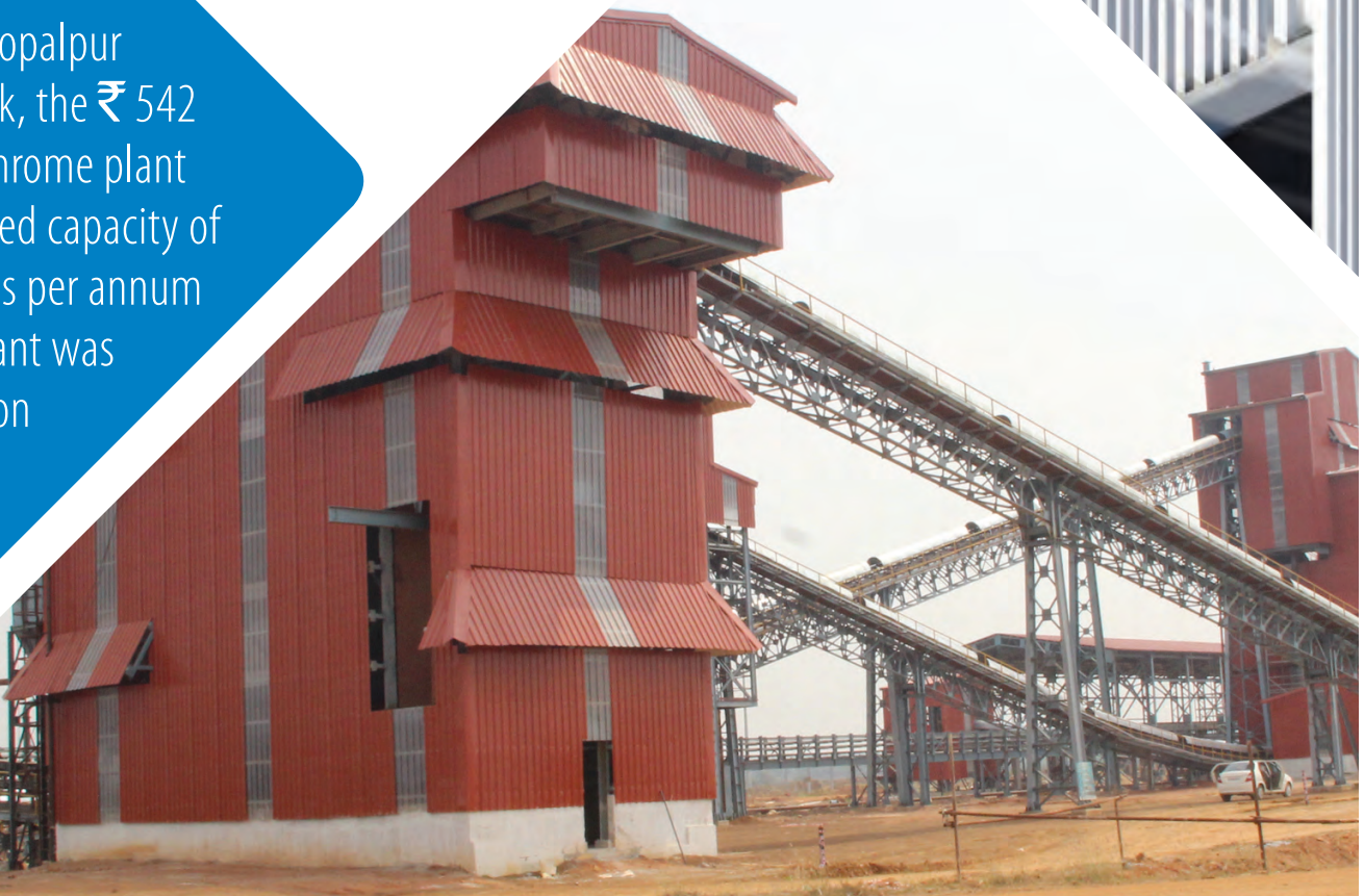
▼ The briquetting plant at Gopalpur
