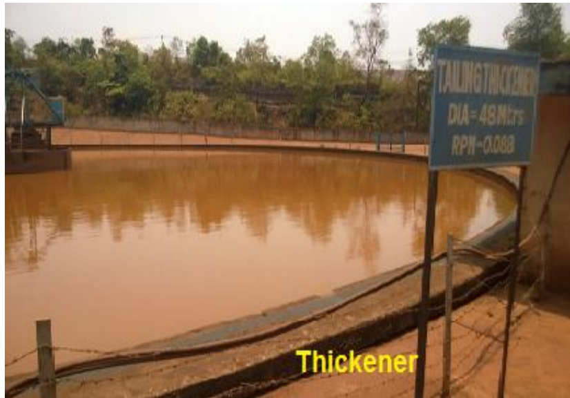
Thickener and Water Recirculation Arrangement
