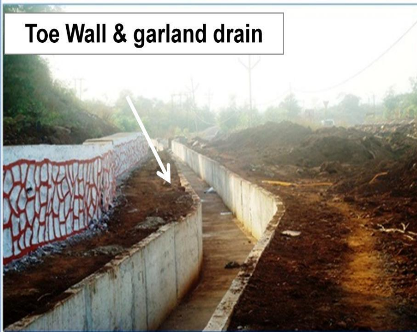
Surface runoff channel
