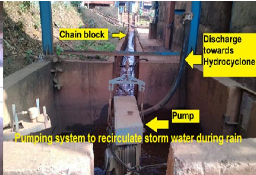
Tailing Dewatering Plant and Water Recirculation Arrangement
