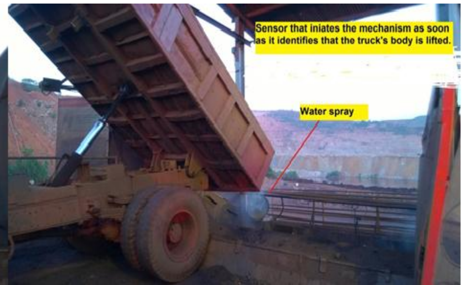
Dust Suppression System at Hopper
