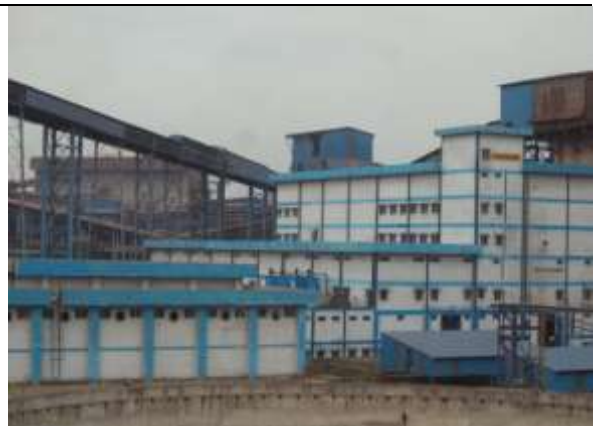
Reverse Osmosis Building
