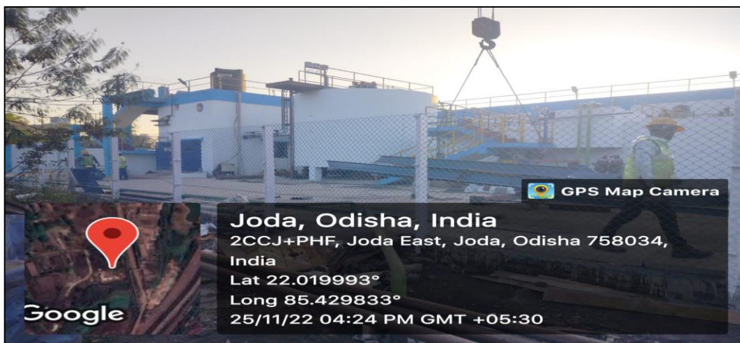
EFFLUENT TREATMENT PLANT (ETP)-30 M3/HR (CONSTRUCTION FINAL STAGE)
